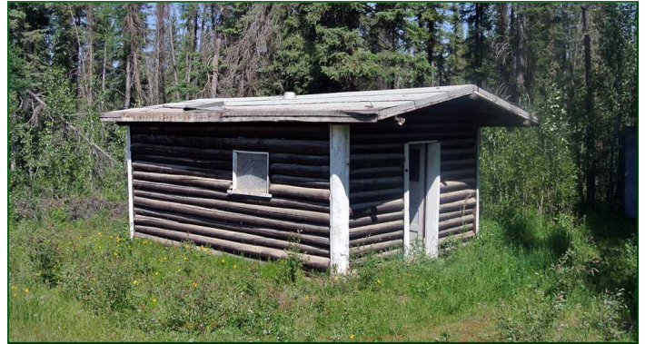
A survival hut on the McKenzie Highway – a life-saver in winter along a stretch of unattended road
